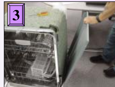
Removing side panels
