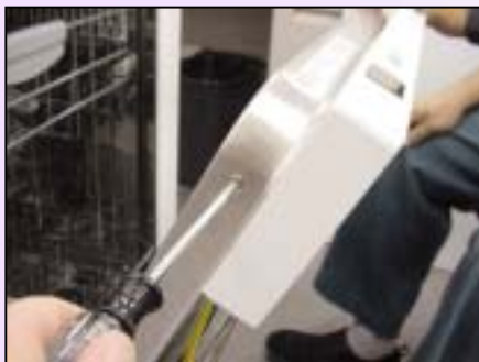
Removing door screws
