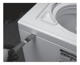
3. Remove two screws retaining Lid Switch.
