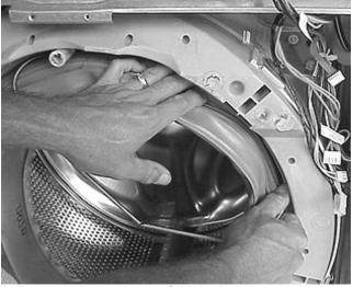
9. Remove the wedge, unfold the bellows, and insert the advance rinsing technology hose .
