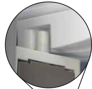
Door Opening - Pin Exiting Track
